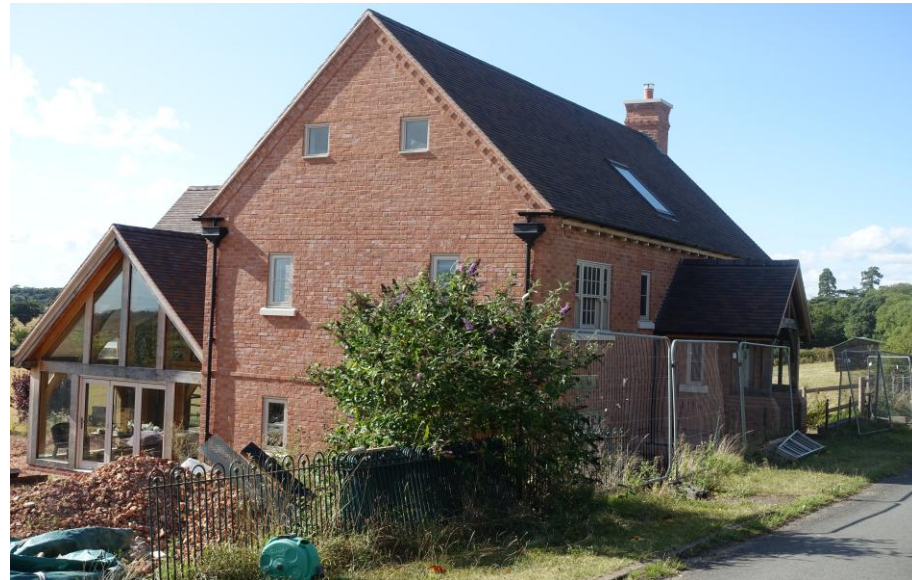
Woodbine Cottage under construction, Walton Hill
