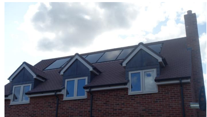
Solar panels being installed into a house under construction in Apperley
